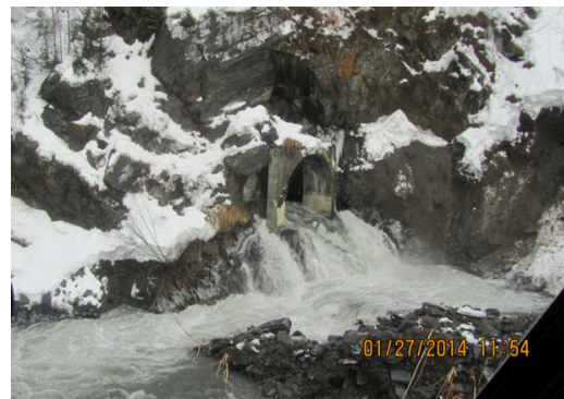
Fig. 5: Old highway tunnel allowing drainage
