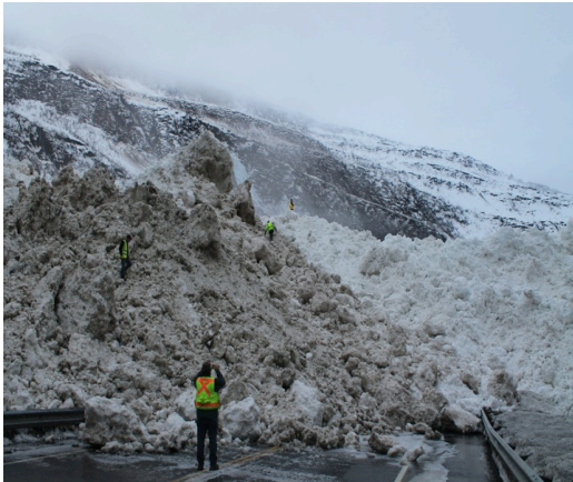
Fig. 4: AKDOT crew surveying Damalanche and buried highway.
